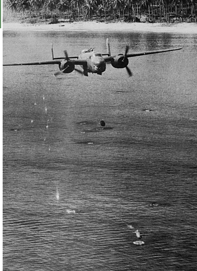
One innovation Kenney engineered was skip bombing, where low flying aircraft skipped bombs across a body of water until they hit the intended target and exploded. Here, a B-25 skips bombs off the water during a run at Wewak, New Guinea.
