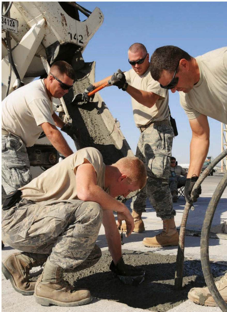
Fill the Hole: 380th Expeditionary Civil Engineer Squadron members SSgt. Robert Hendrickson, SrA. Michael Moulton, TSgt. Gerald English, and TSgt. Bryan Layfield (l-r) pour concrete to build an aircraft tie down at a forward operating location in Southwest Asia. Military civil engineers have served in every major conflict since before World War I.
