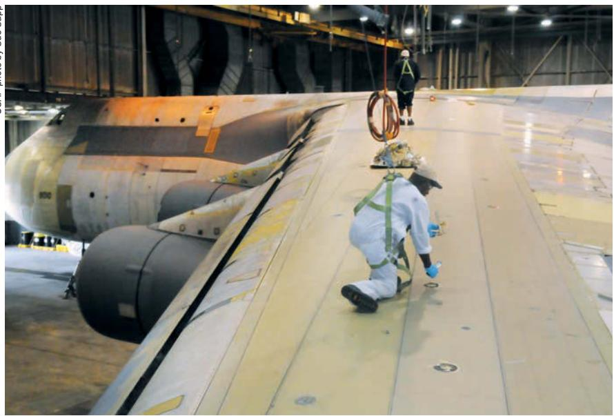
**Painters from the 402nd Corrosion Control Flight prep the wing of a C-5 for the painting process.**
