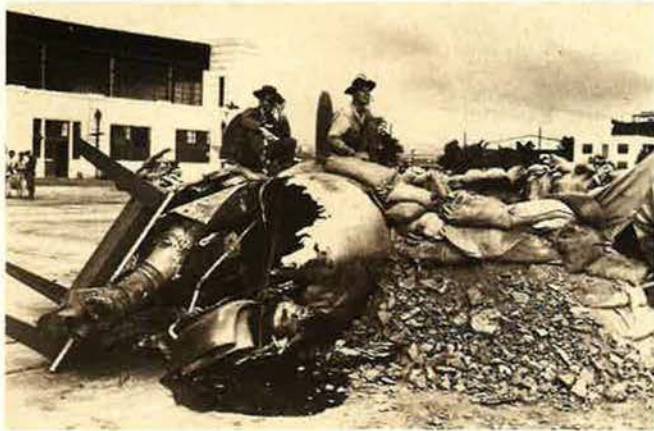
Lieutenant Reid was surprised that his telegram (left) got out on that chaotic day, but the operator took a business-as-usual approach. She was not the only one unaware of Japanese intentions. This makeshift gun emplacement testifies to the unpreparedness of US forces in the region.
