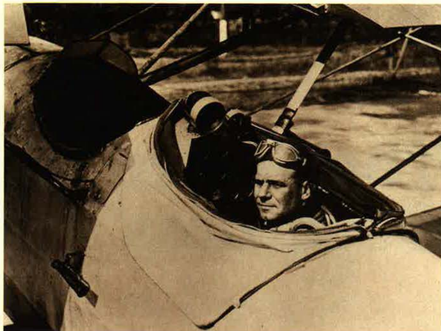
Lieutenant Doolittle prepares for a test flight (note different instruments from those in the preceding picture). To cut off all visual cues other than those provided by instruments, a hood (shown here rolled down) was fitted over the cockpit. Lt. Benjamin S. Kelsey occupied the front cockpit as a safety pilot.
