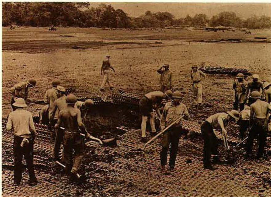
Marston mat's simple design facilitated easy repair as well as easy installation. Locked together by a hook-and-slot design, beaten into the earth with sledge hammers, and secured by steel spring clips, sections of runway could be removed with a pry bar. Here, troops repair bomb-damaged portions of Henderson Field, Guadalcanal.
