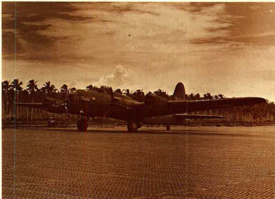
This Marine Corps photo from World War II shows an AAF B-17 Flying Fortress resting securely on a Marston mat runway on Guadalcanal. Basically unchanged some twenty-five years later, the material became known as "PSP," for "pierced steel planking," and hundreds of thousands of tons of it were laid throughout South Vietnam to support far heavier aircraft.
