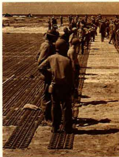
By itself it's not much (right), but stick a few together and you have a well-drained, dust- and mud-controlling, instant runway capable of supporting heavy bombers. This versatile material became the footprint of Allied airpower in World War II.
