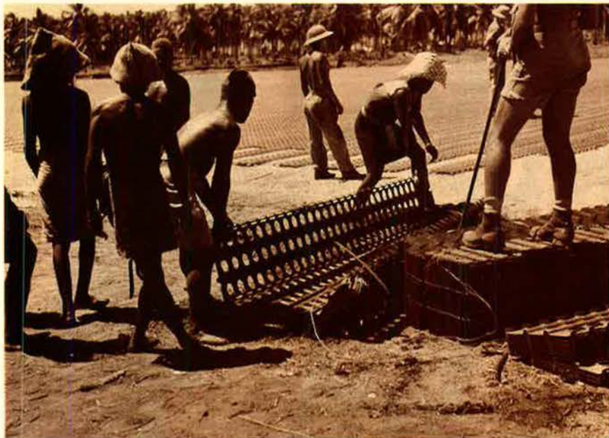
Marston mat's compact dimensions and relatively light weight made it easy to ship and to carry. Wired into bundles and subbundles, 375 square feet of runway surface stood only twenty-eight inches high. Two men could pick up a piece and run with it. Here, a Guadalcanal airfield is improved with Marston mat after the island's capture from the Japanese.
