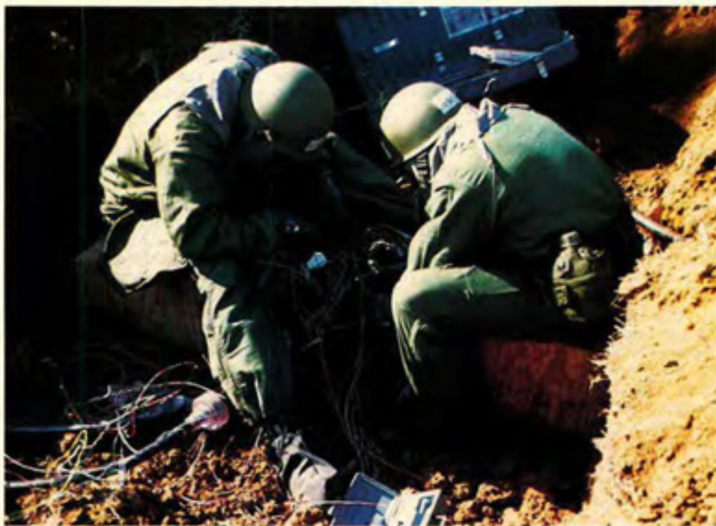
Two members of AFCC's Engineering and Installation Division, wearing chemical warfare suits, practice wartime restoration of communication capabilities for USAF information systems.
