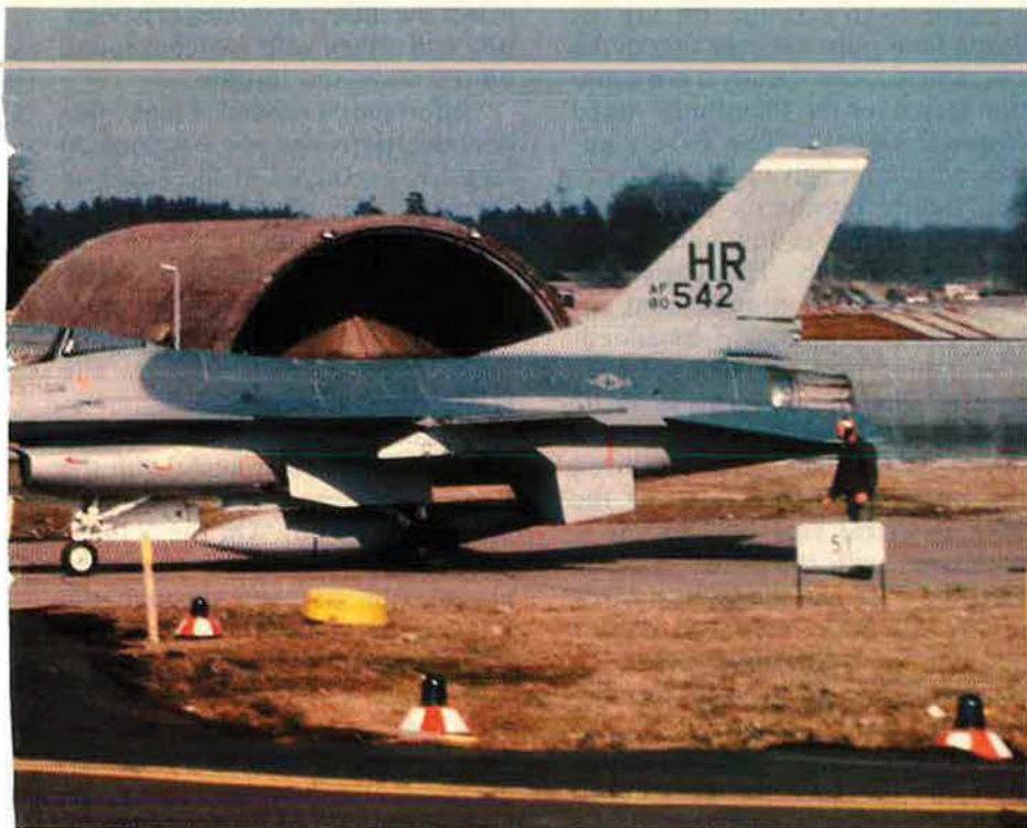
ABOVE: In accordance with NATO's requirement for hardened facilities, TAB-V aircraft shelters have been constructed at Hahn to give its F-16s a measure of protection from aerial attack. RIGHT: As is the policy throughout USAFE, heavy emphasis is placed on performing tasks while dressed against chemical warfare.
