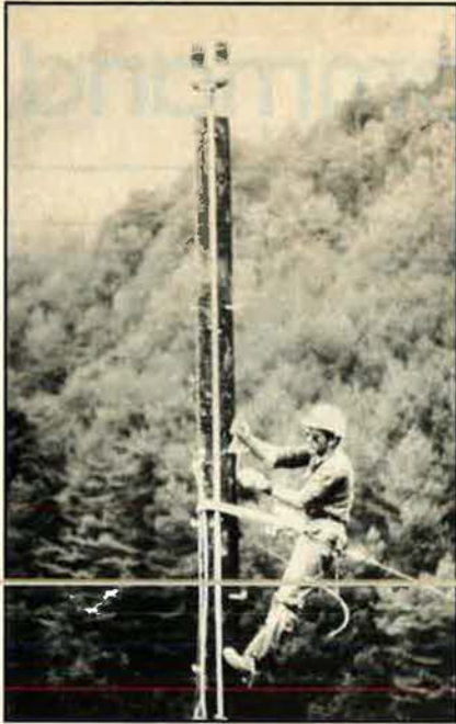
In Korea, Sgt. Robert Foley works on high-frequency antenna during construction of the Korean Tactical Range (Photo by TSgt. Bertram W. I. Mau)
