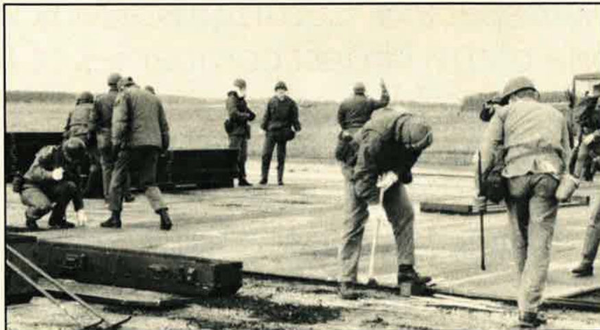
The RAF Bentwaters Rapid Runway Repair Team holds the UK record for laying a fifty-four-foot by seventy-seven-foot mat in sixteen minutes, nine seconds. USAFE is testing the use of concrete slabs instead of conventional aluminum matting as a quicker and more economical method of repairing runway craters.
