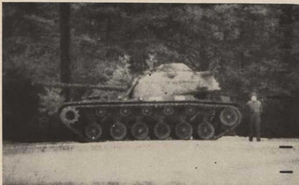
Photo at left was taken through a Starlight Scope on a night so dark that it was impossible to see another person ten to fifteen feet away. As this photo illustrates, the Starlight Scope and other new night-vision devices present the possibility of eliminating the night and allowing troops to operate in "perpetual daylight."
