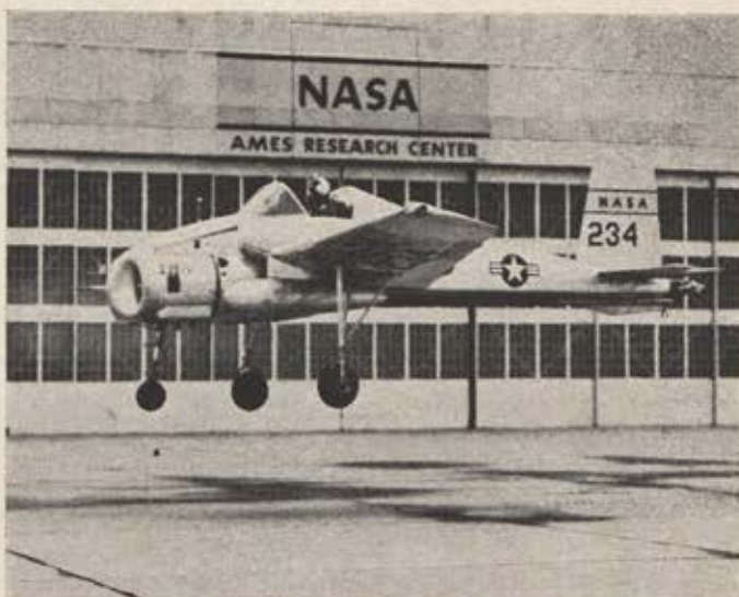
STILL FLYING after ten years, the X-14A used for V/STOL training, including lunar landing approach simulation, and stability and control evaluations, will now enter new programs of variable stability systems research.
