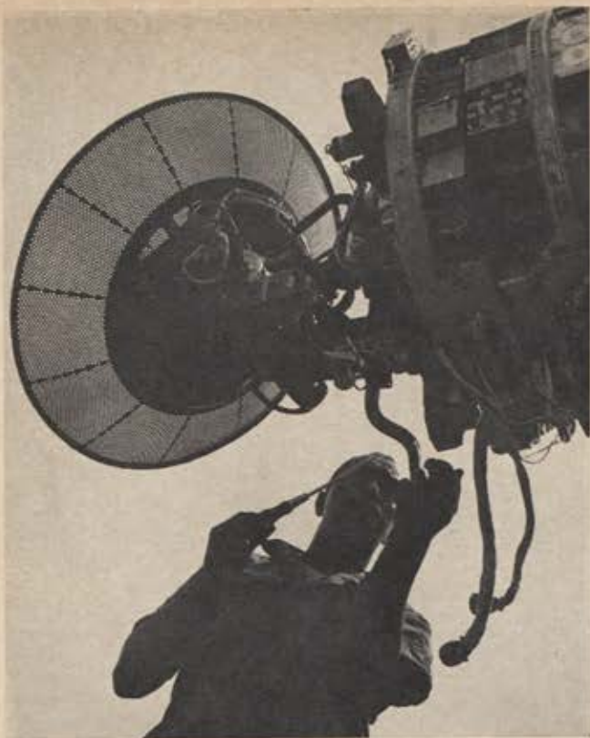
Above, SSgt. Lewis B. Alexander, of Cleveland, Ohio, services the radar set of a supersonic F-4C Phantom II. The radar set on the F-4, most sophisticated and fastest jet fighter in Vietnam, is located in the nose of the aircraft.
