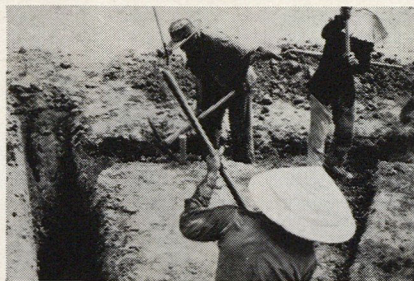
Vietnamese prepare ground to receive Bliss BAK-12 unit.
