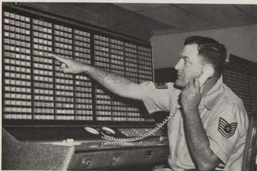
Board which shows condition of 10,000 defense communications circuits simultaneously is operated by TSgt. D. L. Clark, NCOIC of new NORAD-ADC communications outage and restoration section at Ent AFB, Colo. Facility locates and corrects flaws in circuits stretching over sixteen million line miles of NORAD sites in continental US and Canada, and BMEWS net from Alaska to England.
