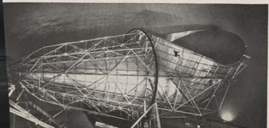
INSIDE GROUND STATION "RADOME" AT ANDOVER, MAINE. Giant antenna (note man near rim of horn) concentrates signals to Telstar in a narrow, powerful beam. The same antenna also receives extremely weak signals coming from Telstar and amplifies them billions of times.
