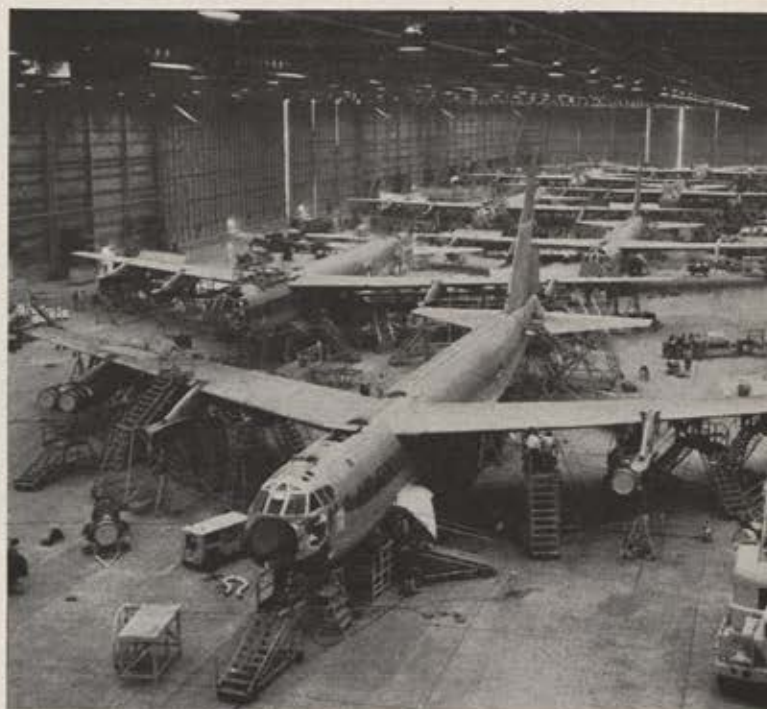
Half of Strategic Air Command's B-52s undergo overhaul and modernization in Aircraft Maintenance Shops at AFLC's San Antonio Air Materiel Area, Kelly AFB, Tex. Thirteen B-52s can be handled simultaneously in this huge hangar at Kelly. The building is 2,000 feet long, 300 feet wide.
