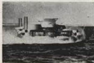
The Bristol Siddeley Viper turbojet currently powers the SR-N1 Hocer aircraft.
