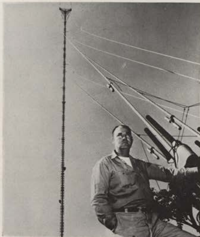
This 1,428-foot high television tower near Dallas, Tex., does double duty as the world's tallest meteorological research structure through a Systems Command contract.
