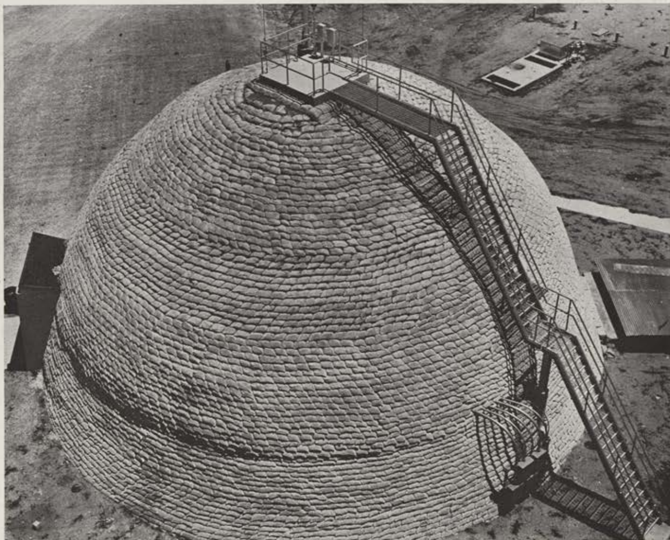
Minuteman ICBM blockhouse covered with sandbags at Cape Canaveral, Fla., an AFSC facility that plays central role in testing of new second-generation, solid-propellant missile. Blockhouse is concrete shell, two levels inside.
