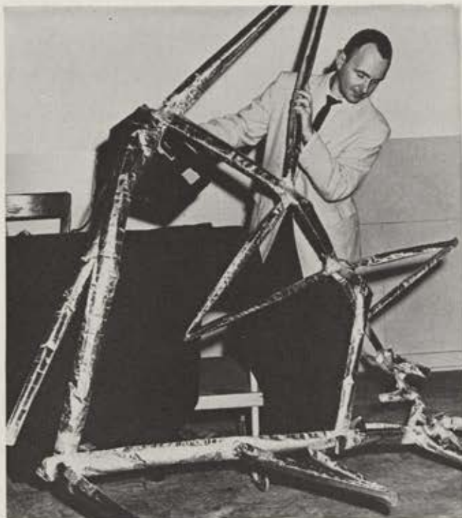
AFSC is deeply involved in space developmental projects. Above, a collapsible antenna proposed for space vehicles.
