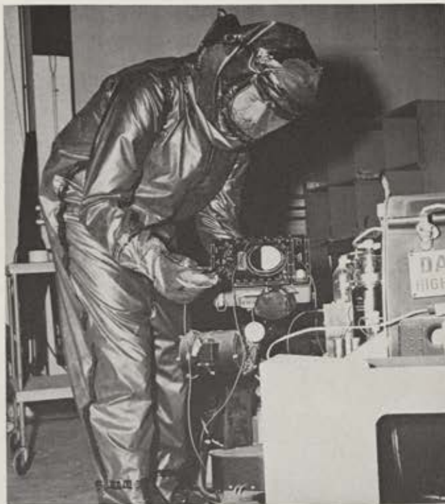
This is not a space suit, but AFSC-developed garb to protect radar technicians working on electronic antennas.
