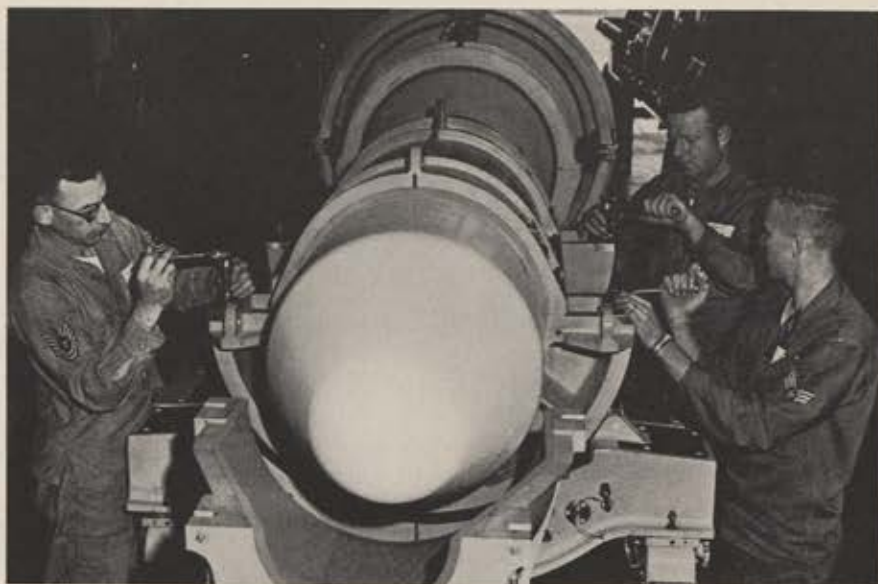
Final assembly of this Mark 3 reentry vehicle is complete and in a matter of hours it will sit atop an Atlas. Here technicians SSgt. Hugh Shelley, Jr., A1C John Lindgren, and TSgt. Arthur Quirk secure vehicle in cradle for trip to pad.
