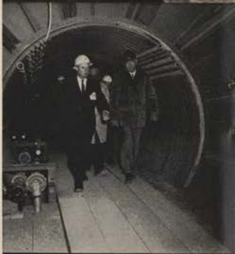
Federal Electric Corporation President, J.W. Guilfoyle (on left), inspects typical underground passageway during initial phase of the complex's activation by FEC.
