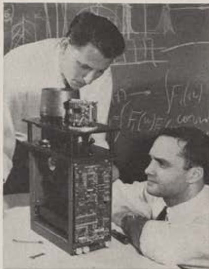
Engineers Harold Sachs and John J. Russo of the Perkin-Elmer Corp. of Norwalk, Conn., examine infrared spectrometer to be carried to Martian vicinity by NASA probe to explore life possibility.
