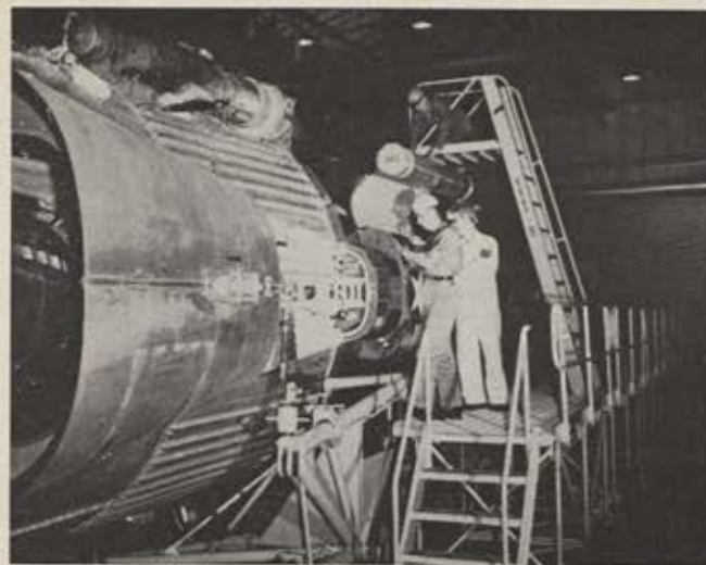
Atlas wiring gets safety inspection from seasoned technician while a student missileman in white coveralls looks and learns. Operational missiles need periodic inspections.
