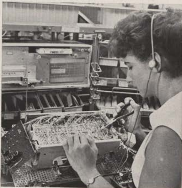
Videosonic Assembly Techniques represent the most important development in line flow since the standard assembly track. This Hughes device regularizes flow, maintains reliability and quality, reduces worker fatigue.
