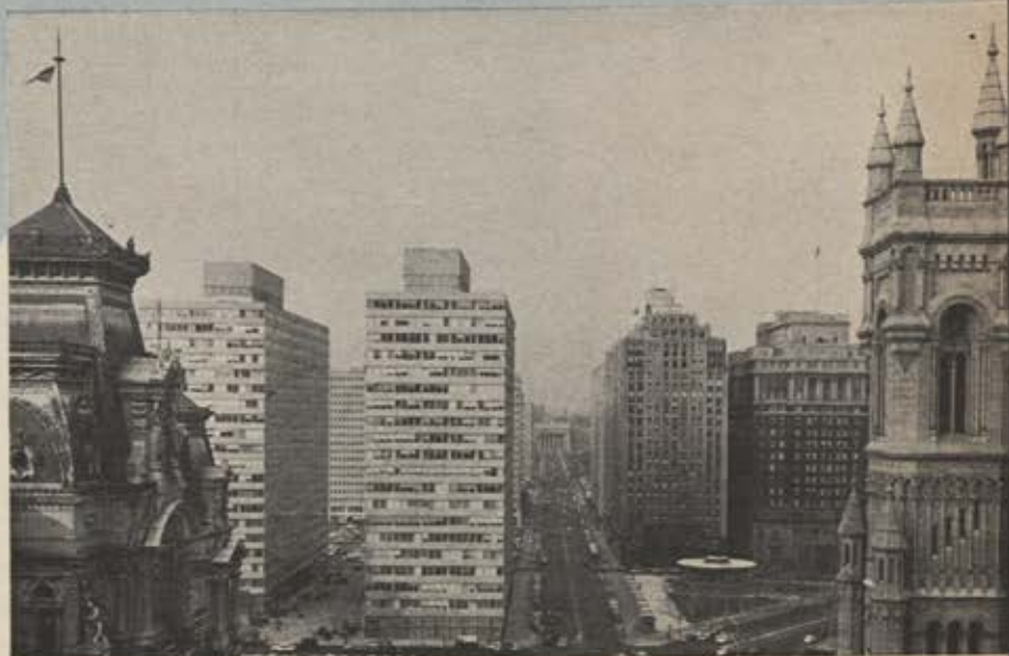
Above: View of "new" Philadelphia's Penn Center area from City Hall to the 30th Street Station.
