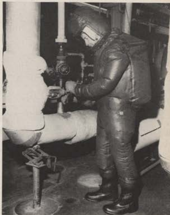
Several lightweight safety suits for rocket-fuel handlers have been developed under Air Force contracts. These suits, weighing from 25 to 30 lbs. with a two-hour supply of liquid air for breathing and air-conditioning purposes are fireproof, moisture proof, and airtight to protect against the inhalation of poisonous chemicals. Adaptations of these suits are being studied to allow relatively unrestricted movement on the moon for a few hours.
