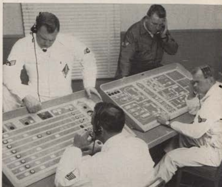
Enlisted technicians hard at work learning to be Atlas missilemen in simulator's control room. At left is model of launch operator's console. Right, second console for missile systems analyst technician, launch troubleshooter.
