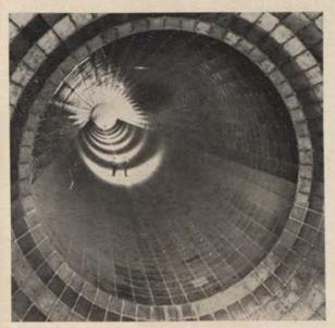
This giant propulsion wind tunnel at Air Force's Arnold Engineering Development Center, Tullahoma, Tenn., is designed for tests of vehicles at speeds ranging from Mach 1.5 to around Mach 5.
