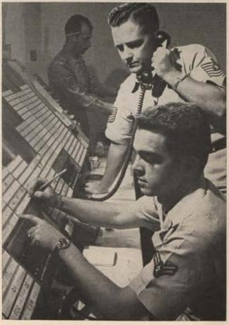
One Caribbean Air Command responsibility is to provide air traffic control in Panama area. Here members of MATS AACS squadron at Albrook man radio, air control boards.
