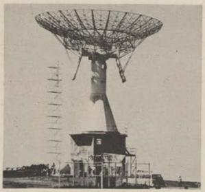
Big ear on Air Force Discoverers is this huge sixty-five-foot-wide parabolic antenna which receives signals from the vehicles during the launch phase and later as they proceed in their orbits.
