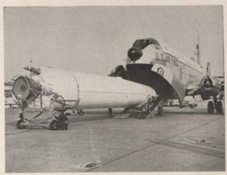
Loading a Thor IRBM into a C-124 transport. Airlift was used extensively in moving Thors to sites in Britain, becomes more and more essential to support modern weapons.
