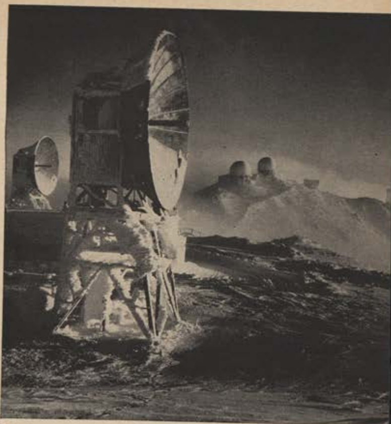
Warning outposts tied to NORAD communications network ring the free world. DEW Line radar stations, one of which is shown above, protect against attack over the top of the world. Station took part in Desk Top III.
