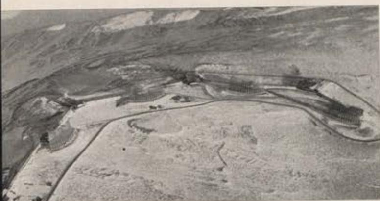
Outside construction is almost completed at Thule. Above, four detection radar antennas, each 400 feet long and 165 feet high. Note rugged Greenland terrain in background.
