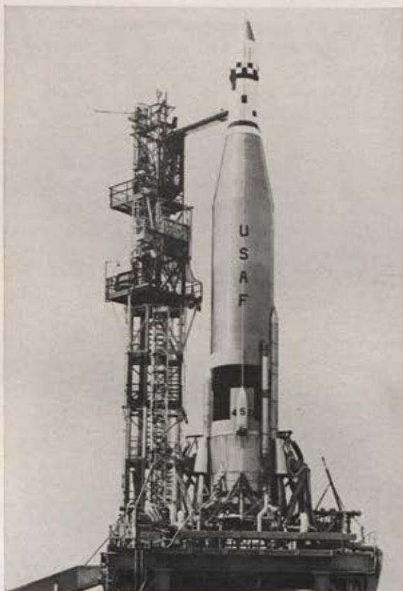
*On pad at Cape Canaveral, Fla., USAF's Midas II infrared early-warning test vehicle awaits May 24 launch into nearly circular orbit. Although orbit was attained, telemetry failure precluded planned test of its capability to detect missile launchings. The orbit did not cross the USSR.*
