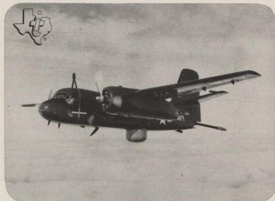
U. S. Navy S2F-1 antisubmarine aircraft, produced by Grumman — equipped with TI-built AN/APS-38A surface search radar, and AN/ASQ-8 magnetic anomaly detector.
