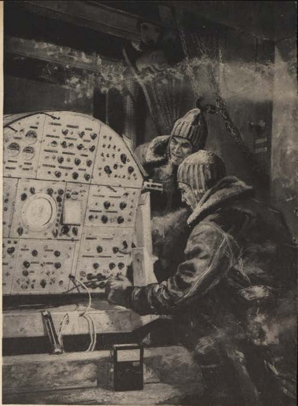
ENVIRONMENTAL CHECK FOR HUSTLER BOMB-NAVIGATION SYSTEM. The USAF's supersonic bomber must maintain global capability over a period of years. Here Sperry engineers put the control console of the B-58's rugged, highly accurate bomb-nav system through its paces.
