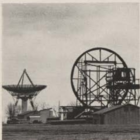
Under construction in foreground is a new antenna which Bell Telephone scientists hope will receive signals reflected from earth satellites during forthcoming tests. Background: a Project Echo transmitting antenna.
