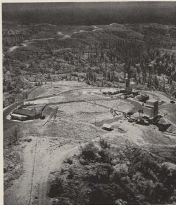
Lockheed's Santa Cruz test facility, seen against rugged wooded mountain area, is remote from new Center. At left, the blockhouse where personnel on scene can handle operations safely.
