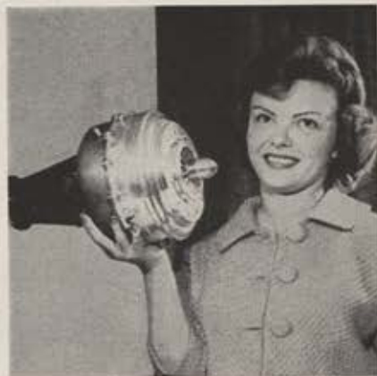
World's smallest turbojet engine, by Williams Research Corp., Michigan, is designed to be mounted on tips of helicopter rotor blades and for other small aircraft use, military and commercial.
