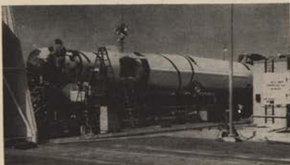
Vandenberg AFB, Calif., engineers at work on the Agena, or satellite stage of a Discoverer vehicle. Boosted by AF Thor IRBM, Agena stage is injected into polar orbit. NASA will be using Agena soon.
