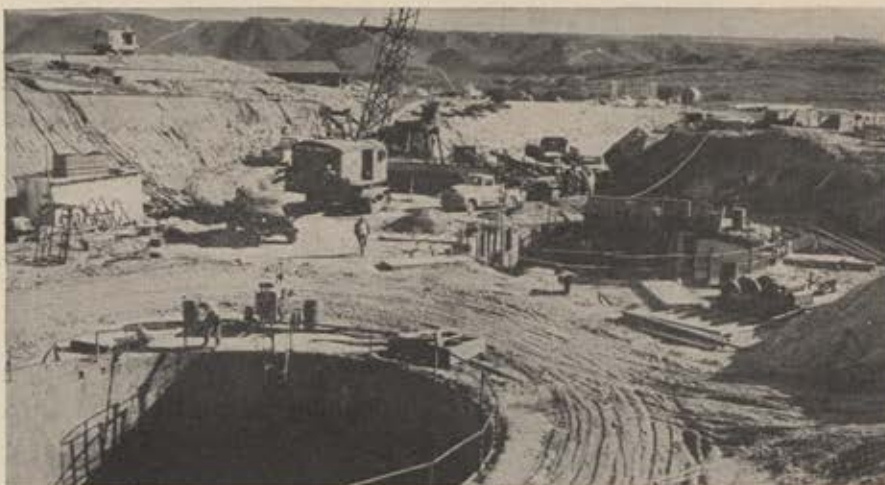
Construction is proceeding on the intricate launch and storage complex for Titan, Martin-built ICBM backup to Atlas. This scene is at Vandenberg AFB, Calif. Army Corps of Engineers builds the silo-like structures for USAF.
