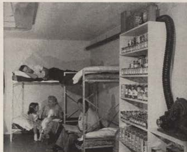
Somewhat luxurious family shelter built under front terrace of $50,000 Pittsburgh home. Total cost was $2,900. Ceiling, walls are concrete. It includes an escape tunnel.
