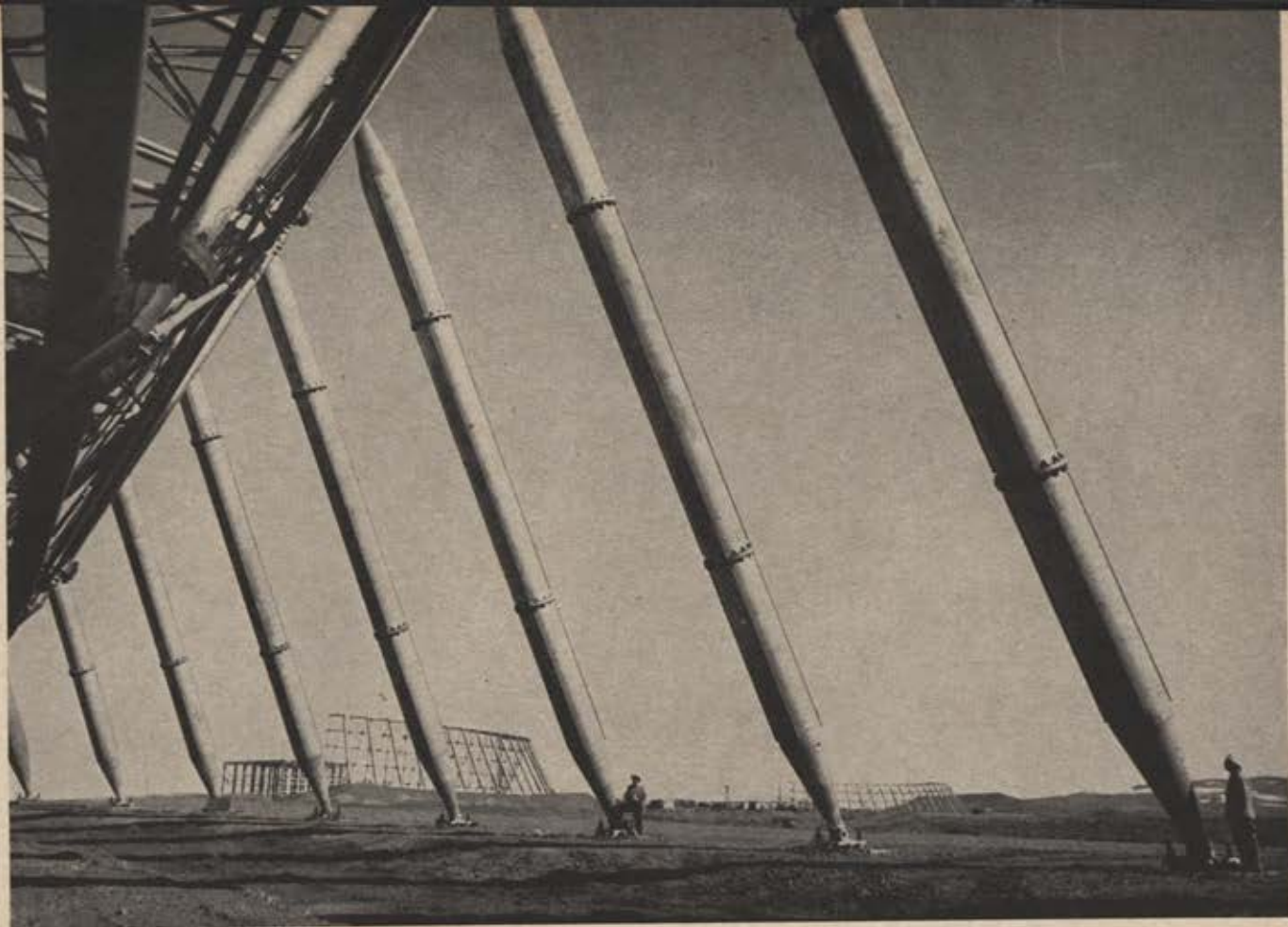
Workmen high in the Arctic are dwarfed by the giant backstays that hold one of the BMEWS antennas firmly in place against winds up to 185 mph. The electronic network is being built to warn against incoming enemy ICBMs. Other BMEWS facilities to warn against enemy missile attacks from the east or west could be located on our overseas bases.
