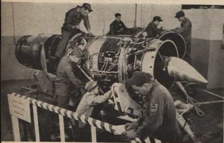
General Electric J-73 jet engine undergoes maintenance at USAF base. Such daily tasks grow increasingly complex.
