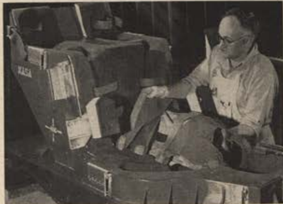
NASA technician works on construction of form-fitting contour couch for Mercury program. Astronauts will have individually molded seats.
