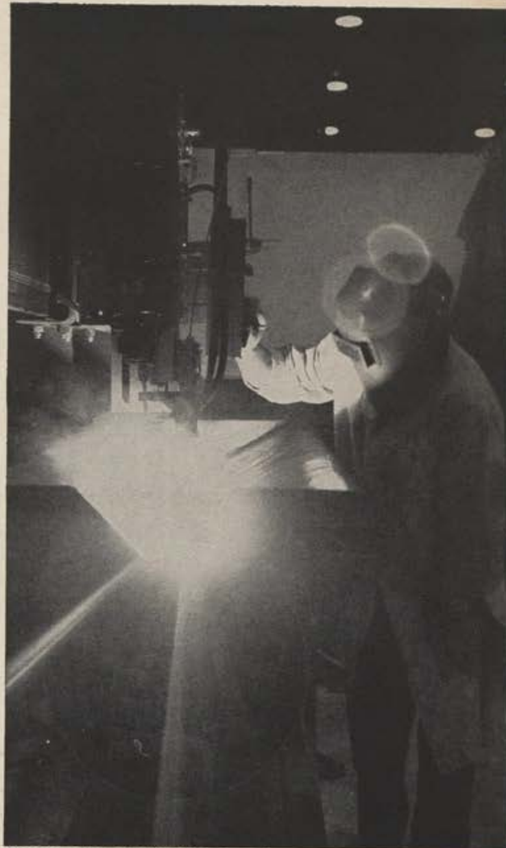
AUTOMATIC EQUIPMENT: Use of automatic equipment like the welding machine above at the Ordnance Department gives time savings of 6 to 1 over manual methods. Automatic machinery also assures uniform high quality and low costs.
