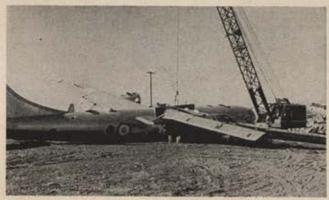
"Guillotine," huge razor-sharp blade wielded from crane, slices neatly into fuselage of old B-29 Superfortress. This one served for period with Britain's Royal Air Force.
