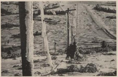
MDA personnel provide communications-electronics support continuously in Far North. Here, in typical Alaskan scene, AC&W site cables snapped by heavy ice.
