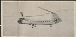
The four-ton H-16, first in Vertal's series of turbinepowered helicopters, flown in 1955.
