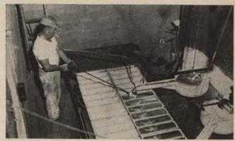
Next step after the knife is the "sweater," or melting furnace. Then the reclaimed metals are sold on the open market. Here melted aluminum is poured into row of ingots.
