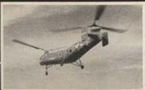
The H-21D research aircraft equipped with two GE T-58 turbo-shaft engines, flown in 1957.
