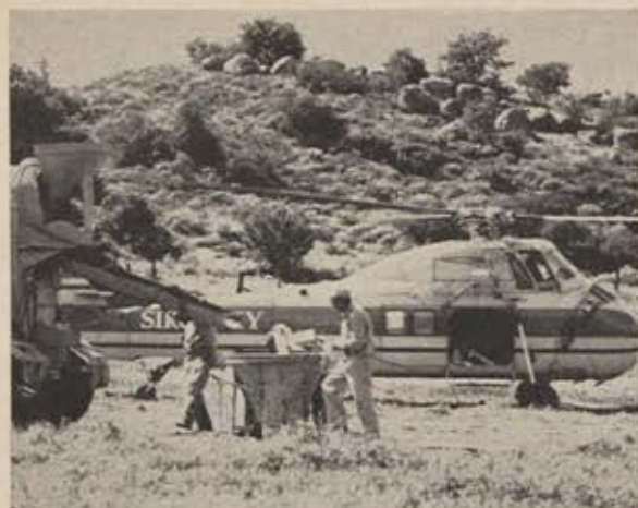
Helicopter is already demonstrating varied capabilities in numerous civilian projects such as oil exploitation, construction, laying power lines in rugged terrain. Here a Sikorsky S-58 helicopter plays major role in setting up transmission towers in California hills. Left, S-58 picks up hopper at mixer miles from tower site. Center, 'copter carries hopper over mountains to building crews. Right, S-58 hovers, drops cement for tower footing.
