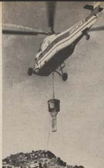
Helicopter is already demonstrating varied capabilities in numerous civilian projects such as oil exploitation, construction, laying power lines in rugged terrain. Here a Sikorsky S-58 helicopter plays major role in setting up transmission towers in California hills. Left, S-58 picks up hopper at mixer miles from tower site. Center, 'copter carries hopper over mountains to building crews. Right, S-58 hovers, drops cement for tower footing.
