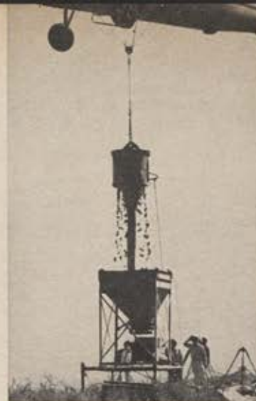
Helicopter is already demonstrating varied capabilities in numerous civilian projects such as oil exploitation, construction, laying power lines in rugged terrain. Here a Sikorsky S-58 helicopter plays major role in setting up transmission towers in California hills. Left, S-58 picks up hopper at mixer miles from tower site. Center, 'copter carries hopper over mountains to building crews. Right, S-58 hovers, drops cement for tower footing.
