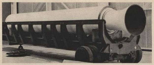
Solid-fuel rocket developed by Aerojet-General as the first stage of Project Scout, NASA's "poor man's rocket."
