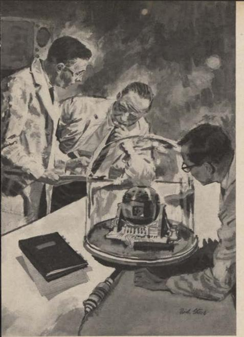
TO GUIDE USAF'S B-70 SUPER BOMBER — Sperry-developed Rotorace™ gyroscope (being tested in laboratory) is heart of Sperry Twin-Gyro Platform which will help crews hold accurate course in any weather, day or night, at any point on earth.
