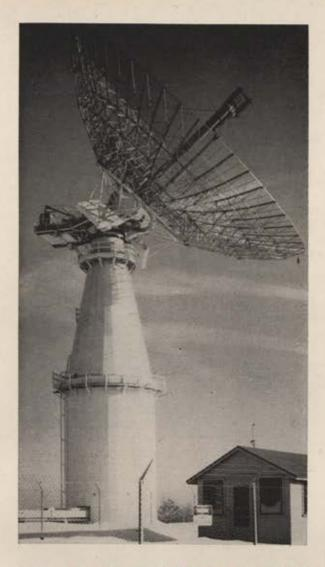
Lincoln Laboratory's Millstone Hill radar used in bouncing round trip radar to, from Venus.
