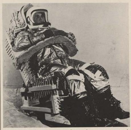
Resting comfortably, an Air Force researcher tests the prototype net system designed to support body in high-altitude acceleration during rocket-powered flight.
