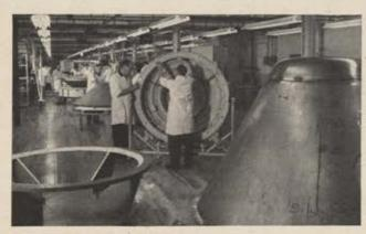
RE-ENTRY VEHICLES ARE ASSEMBLED at MSVD facilities in Burlington, Vt., for both THOR and ATLAS ballistic missiles.
