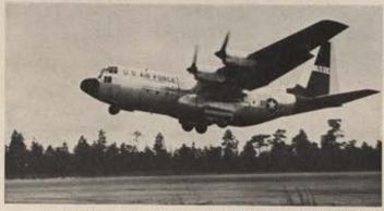
Takeoffs from deep sand averaged only 1500 feet in a C130A at 110,000 pounds gross weight. With same load it landed on sand and stopped in less than 950 feet.
