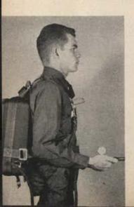
USAF is studying possibilities of providing weightless spacemen with personal locomotion devices. Pack of compressed air cartridges is used to determine amount of gas pressure needed to move a man in controlled direction. Finished device might look somewhat like a hand reaction "gun."
