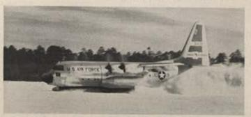
Landing on frozen lake, "Ski-130" (weighing 62 tons gross) stops in 1200 feet. Taking off from same lake, this ski-fitted Airlift Champion was airborne in 2100 feet.
