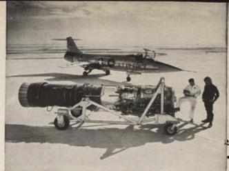
GENERAL ELECTRIC FLIGHT PROPULSION ACHIEVEMENTS include the J79 jet engine, now being built by the Flight Propulsion Division. J79 recently powered USAF F-104 to world speed, altitude, and climb records.
