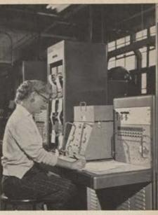
AUTOMATIC FUNCTION SIMULATOR, one of the newer testing techniques used by Westinghouse, assures more reliable protective devices for electrical systems. This machine subjects protective control panel to as many situations as it will encounter in flight operations.
