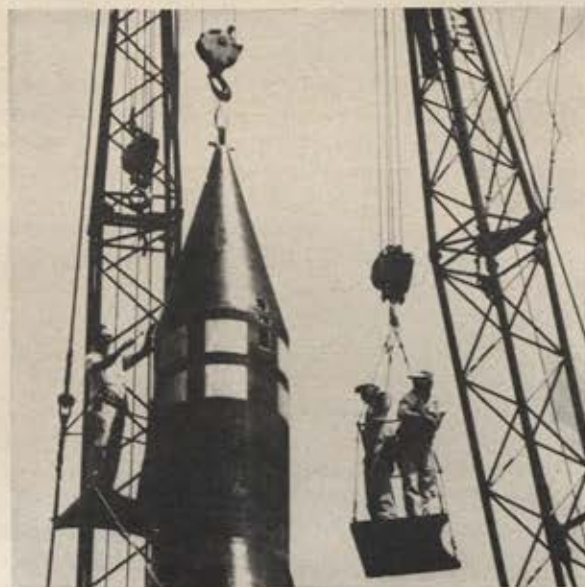
Juno II, US Army space probe vehicle that carried the Pioneer III one-fourth of the way to the moon on December 6 under NASA supervision. The shroud protected the upper stages from atmospheric heating.
