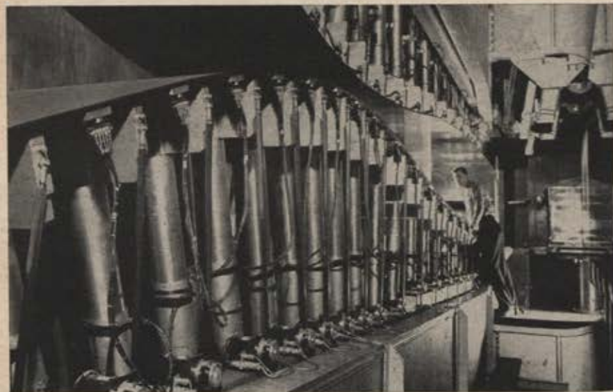
With sidewall removed on Gas Dynamics Facility tunnel, hydraulic jacks may be seen. They change curvature of the nozzle to permit varying airspeeds.
