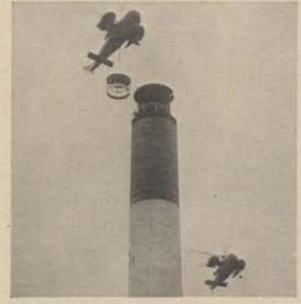
LIFTING THE LANTERN—An HR2S-1 (Sikorsky S-56) from the Second Marine Aircraft Wing places a 1740-lb. lantern atop a new 142-foot lighthouse at Cape Fear, N. C., with only 6 inches of clearance on the sides. Hovering stability for this difficult job was provided by Sikorsky's Automatic Stabilization Equipment in the HR2S-1.
