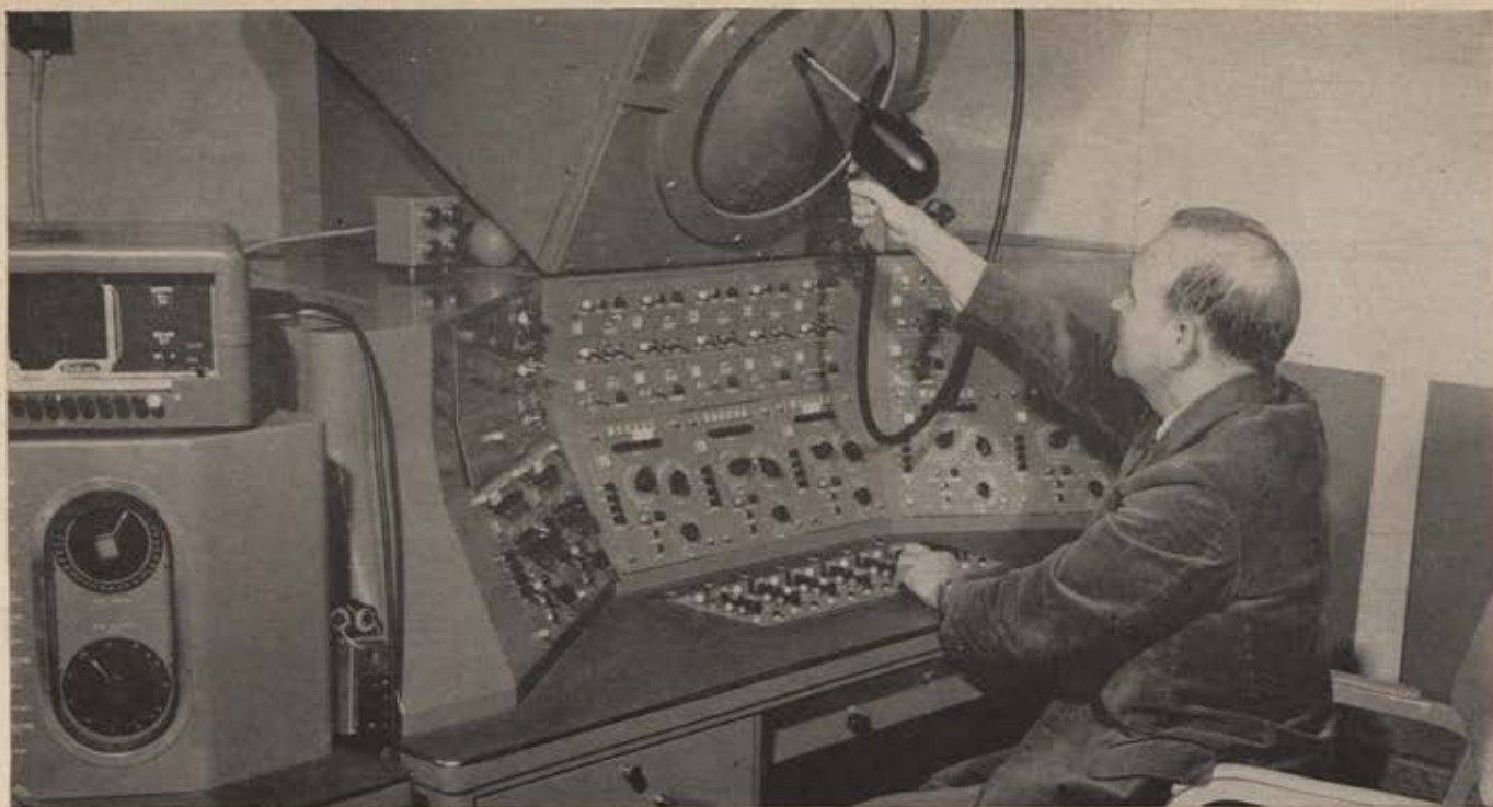
Scientist operates Cambridge-developed light gun used in the VOLSCAN air traffic control system. Use of the gun puts on aircraft "blip" under control of a computer which directs the aircraft to a timed landing under all weather conditions.
