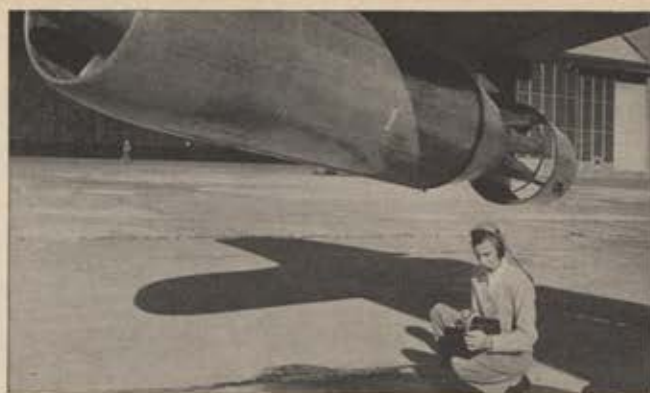
Experimental nozzle shapes to suppress turbojet noise are mounted on a J-47 engine of a B-47 Stratojet for tests.
