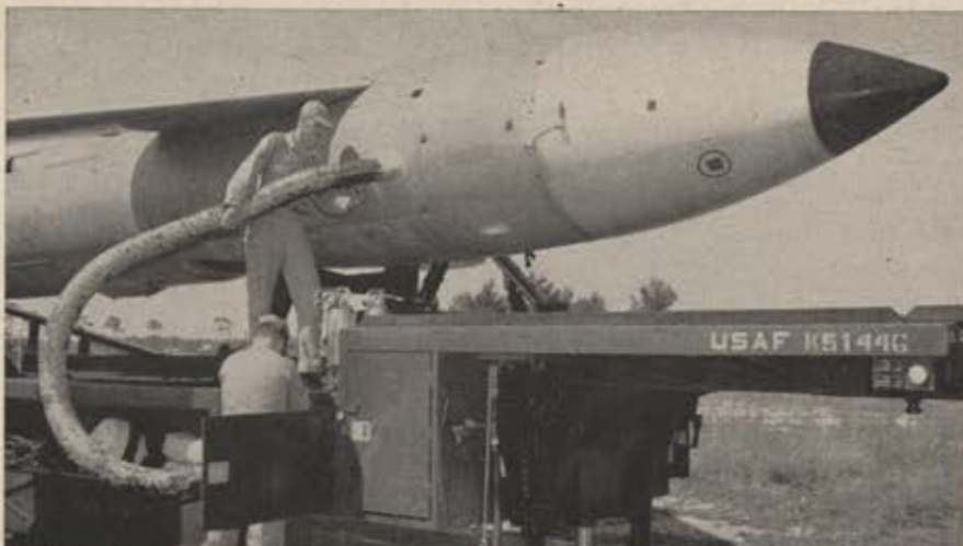
Technicians disconnect the exhaust hose from the TM-61C Matador missile before launching at Patrick AFB, Fla. Hose cools missile electronic components.
