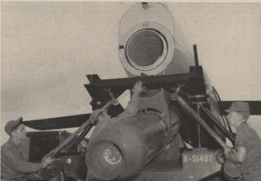
Armament technicians at Patrick connect the RATO unit to the Matador missile. RATO is a rocket booster used to accelerate the missile in initial flight.
