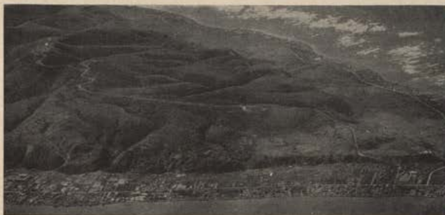
Russian pilot's view of Wakkanai. At lower right, camp, upper left, the radar.
