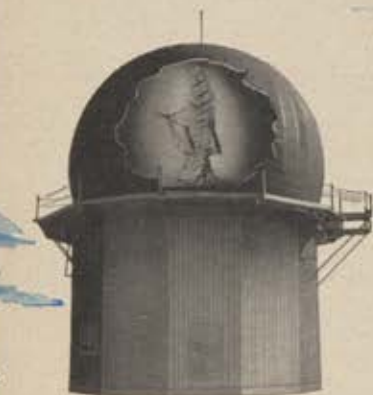
FPS-6 fixed installation in air- supported radome for protection against severe winds, snow and ice.
