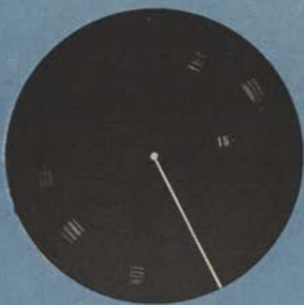
BEACON INTERROGATION: Pilot can orient himself from ground and airborne radio signals. Above, coded signals from six airfields.
