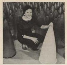
Nose cone for guided missile is made of Pyroceram, a crystalline material developed by the Corning Glass Works.
