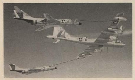
F-101 Voodoo fighters refuel from new KB-50J tanker modified by Hayes Aircraft Corp. with two J-47 jet engines to increase the refueling speed of the tanker.
