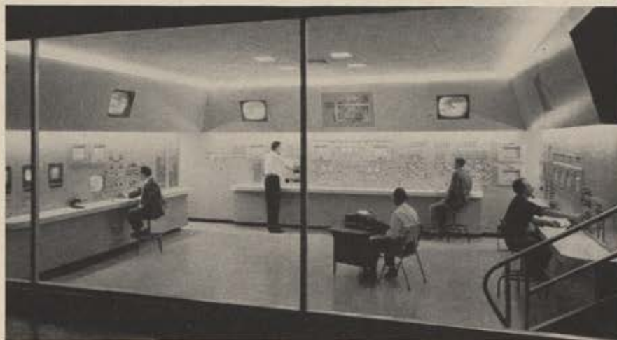
Television monitor sets (near the ceiling) are used in closed-circuit hook-up in the control room of the Lewis Unitary Plan Wind Tunnel, Cleveland. The sets can be connected to any of the three TV cameras that survey the tunnel.
