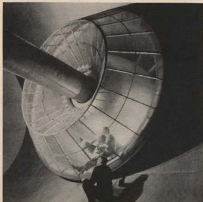
NACA technicians at Lewis Flight Propulsion Lab, Cleveland, check screened inlet of one of the wind tunnel compressors used when tunnel is operated at Mach 2.5 to 3.5.
