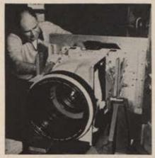
New eye for the AF—a 36" f/4.0 Perkin-Elmer lens gets final adjustment.
