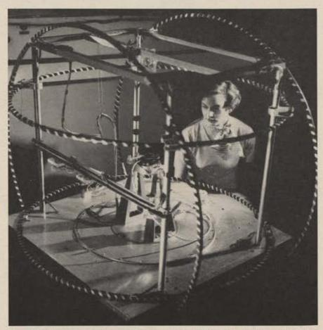
General Electric's test device simulates banking, pitching, and complete turns of aircraft, and it also duplicates the magnetic field of any point on earth. Dark object (center) is part of a highly sensitive compass system under test.
