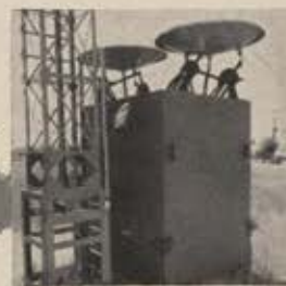
Microwave System capabilities include the transmission of voice communications (up to 72 two-way channels), radar data and radar control functions.
