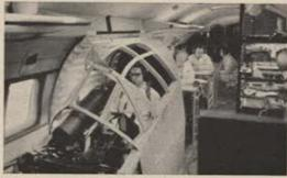
F-102 mock-up in a T-29 permits pilot to test fighter's electronic control system in flight,
