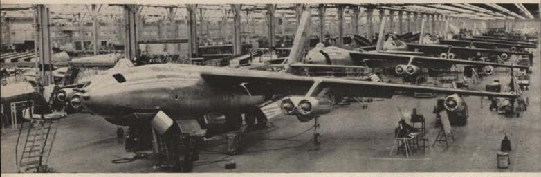
Parallel lines of B-47s stream toward military service at GAP-6. At left: new Lockheed-produced planes. Right: Mod-IRAN line
