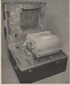
T-11 Camera manufactured by Fairchild Camera and Instrument Company travels safely in water-tight, air-tight case of Koch molded Fiberglas.
