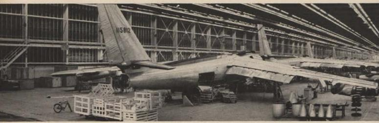
**Side by side,** new Lockheed C-130 Hercules planes (right) and Boeing-designed B-47 Stratojet bombers move along assembly lines
