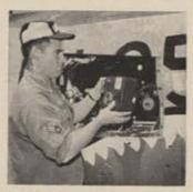
A/2C Thomas Ferguson installs tape-recording NADAR unit in airplane (see text).
