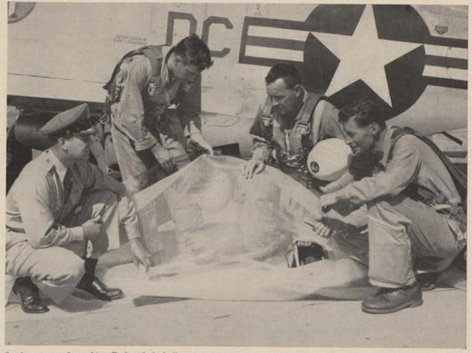
Scoring target sleeve hits. Each pilot's bullets are dipped in a different colored paint which marks the sleeve.
