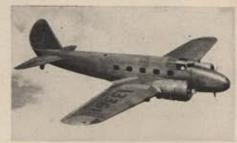
1932 The 247, first 3-mile-a-minute airliner, set basic design for all modern twinengine transports.
