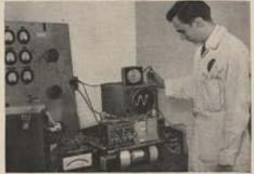
FORD ENGINEER checking voltage and frequency accuracy of power supply unit under simulated load conditions in a project for the Guided Missile Development Division of the Redstone Arsenal.
