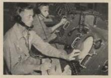
Technicians mark radar scopes to help controller read and evaluate picture.
