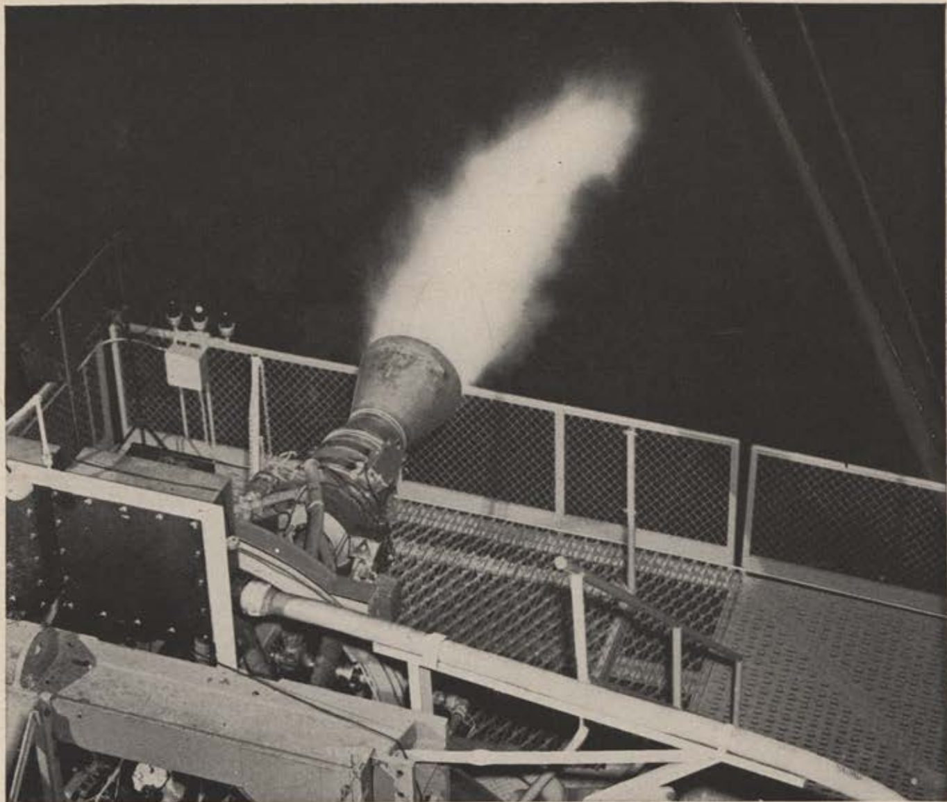
Night firing tests on early ROCKETDYNE engines helped speed the development of today's models whose power cannot be disclosed.
