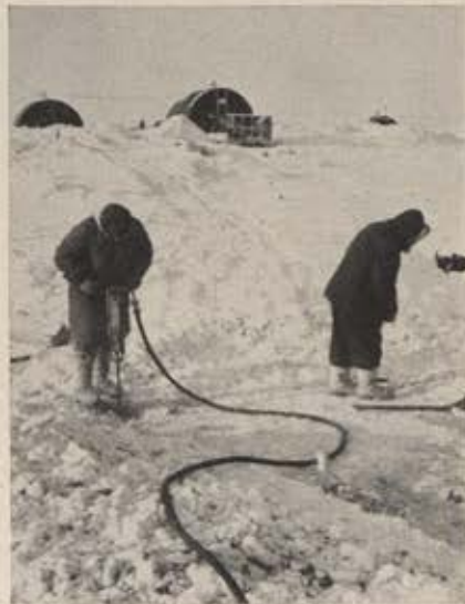
Construction workers drill holes for a foundation on a Baffin Island site.
