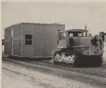
A module is towed to storage area to await transportation to the DEW line.
