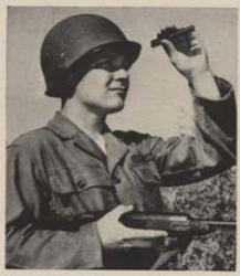
Small Signal Corps dosimeter, built for field use, gives a quick reading of any deadly gamma rays in the area.
