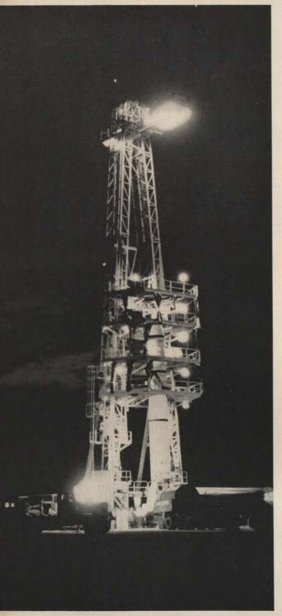
The Army's intermediate range ballistic missile, the Redstone, being fueled and checked in a service tower at Patrick AFB, Fla. The Army considers missiles "artillery."
