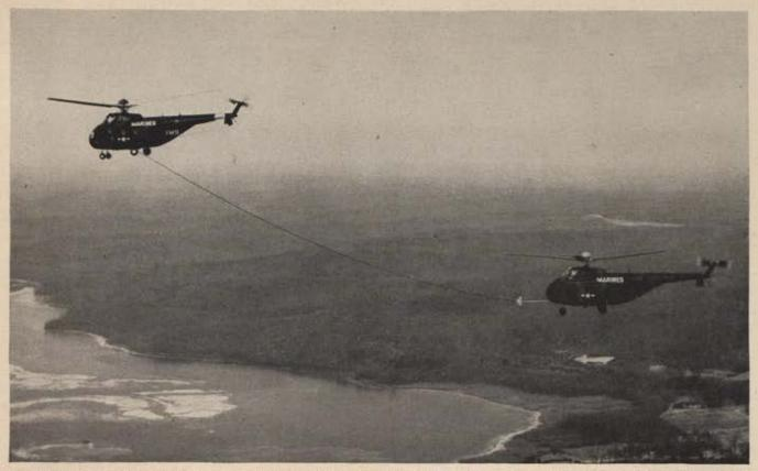
IN-FLIGHT REFUELING technique for helicopters is demonstrated for the first time by two Marine Corps Sikorsky HRS helicopters. By increasing potential range and pay-
