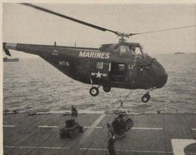
AIRBORNE BULLDOZER —Flying from the escort carrier USS Siboney , a Marine Corps HRS helicopter lifts a bulldozer during exercises in the Atlantic. The HRS is a version of the Sikorsky S-55, used all over the world in industry, in passenger, cargo and mail service, and in many armed forces.
