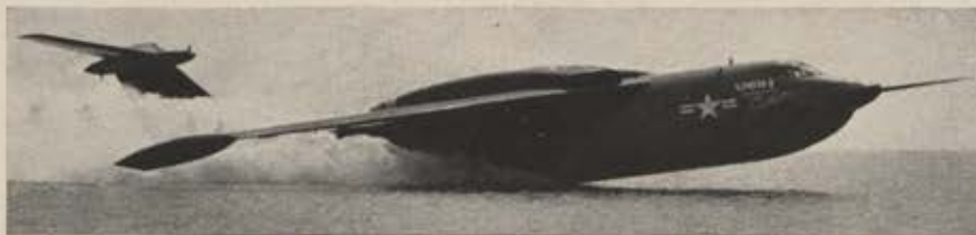
Martin XP6M-1 SeaMaster. Navy says flight tests of 600-mph jet seaplane are "unusually promising." Note wing-top nacelles, wing-tip floats and "T" tail.
