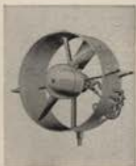
AIR-DRIVEN HYDRAULIC PUMP
