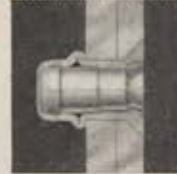
dimpled sheet, 100 degree countersunk head.
