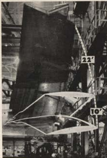
In a test of strength, a Boeing B-52 wing was deflected to these extremes.
