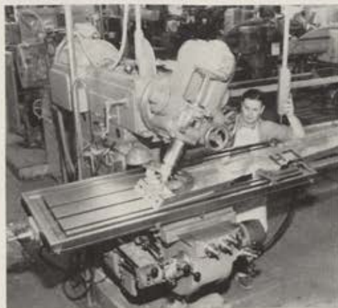
Twin Coach Aircraft Division plants turn out wing spars, main wing panels, flaps, complete center sections with plumbing and electrical wiring, and other large assemblies.
